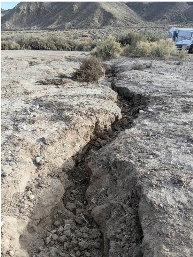
Picture 6-7: Significant channelization and erosion at major staging area leading into closure.
