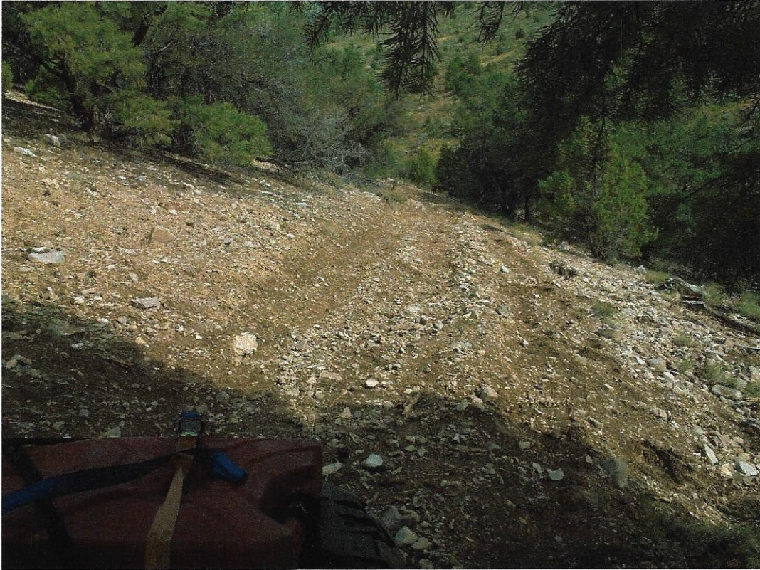
Ranger Trail North of Berry Creek (Note the out-slope which is a safety risk for rollover)
