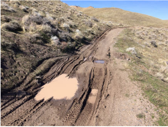
Route 21-520. Example of inadequate drainage.
