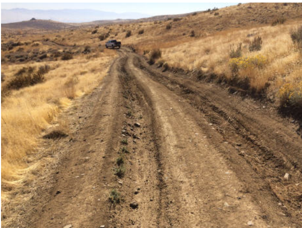
Route 41-652. Needs drainage improvement and removal of ruts.
