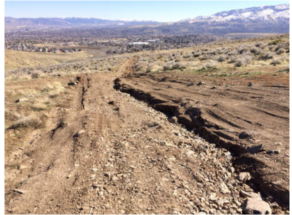
Route 21-520. Example of rutting caused by water not being able to drain off of trail.
