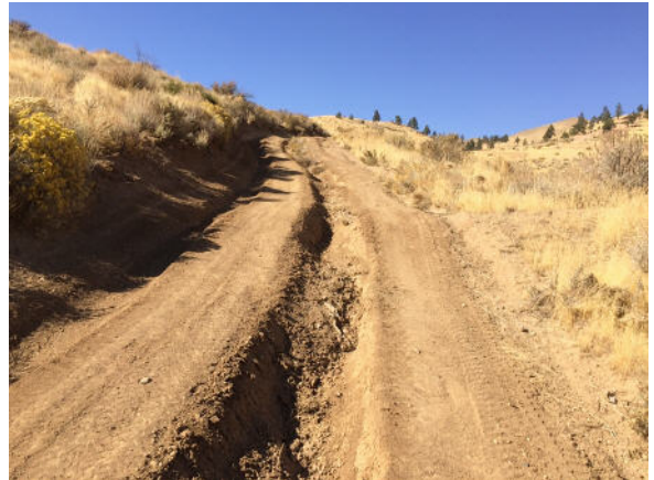
Route 41-649. Needs drainage improvement and removal of ruts.
