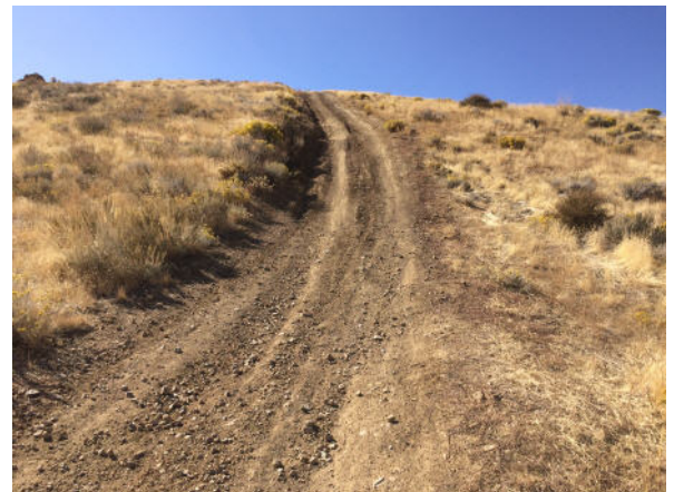
Route 21-535. Needs drainage improvement and removal of ruts.
