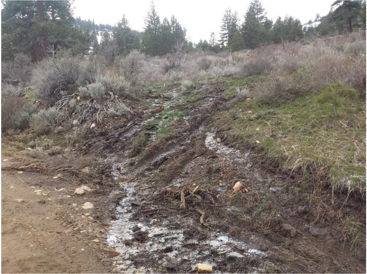
Photo 3: Resource damage from motorists circumnavigating sections of damaged road.
