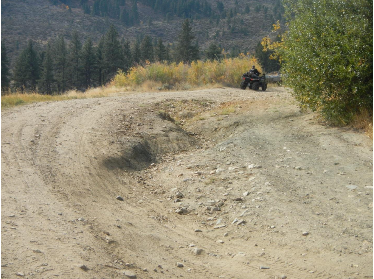
Photo 5: Extensive channeling in the road has resulted in widening of the road as motorists by-pass the damage.
