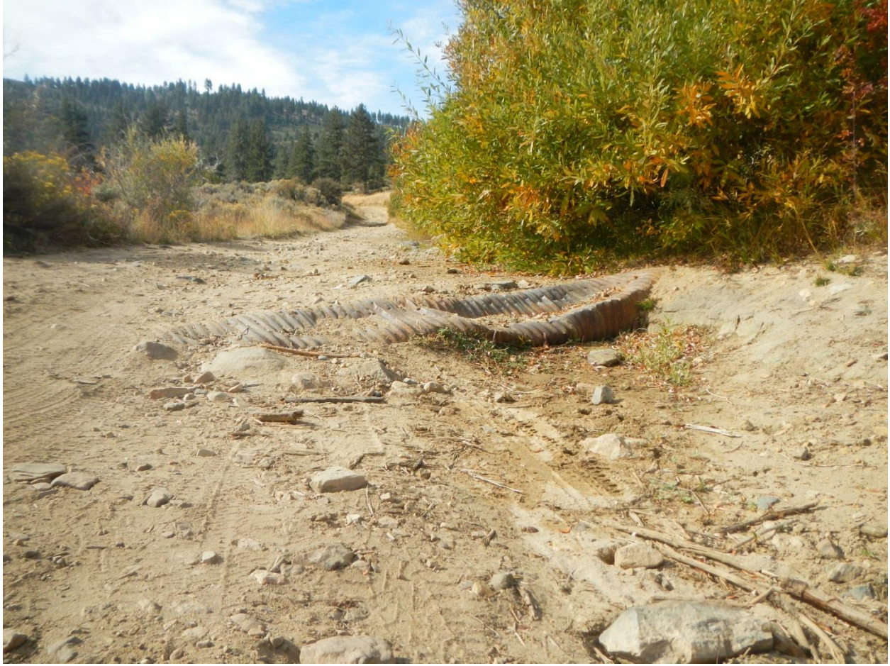
Photo 6: damaged and non-functional culvert.
