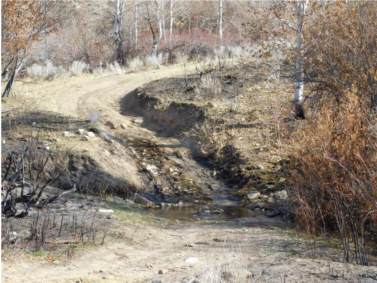
Photo 1: Stream crossing requiring maintenance.
