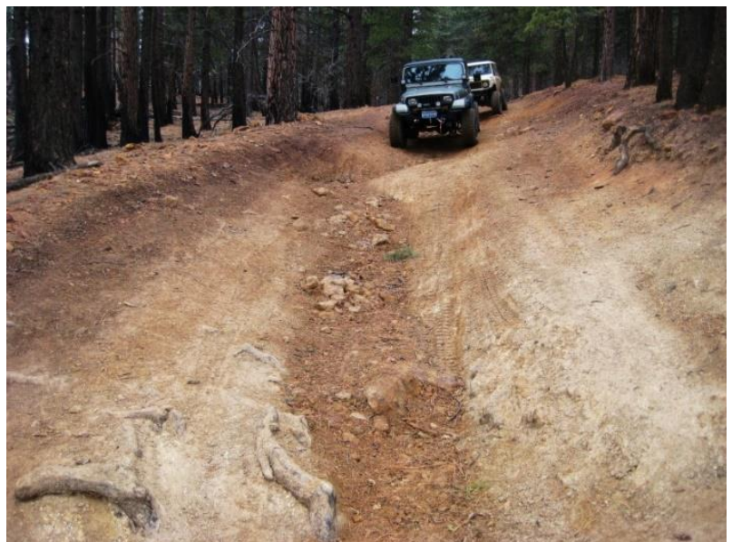
Photo of Hunter Lake road erosion damage.
