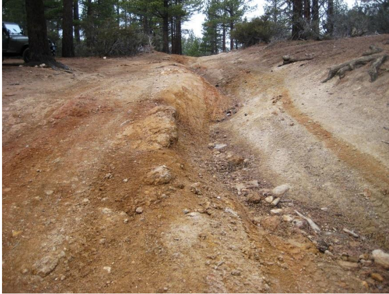
Photo of erosion cutting at the roadbed on State Line road
